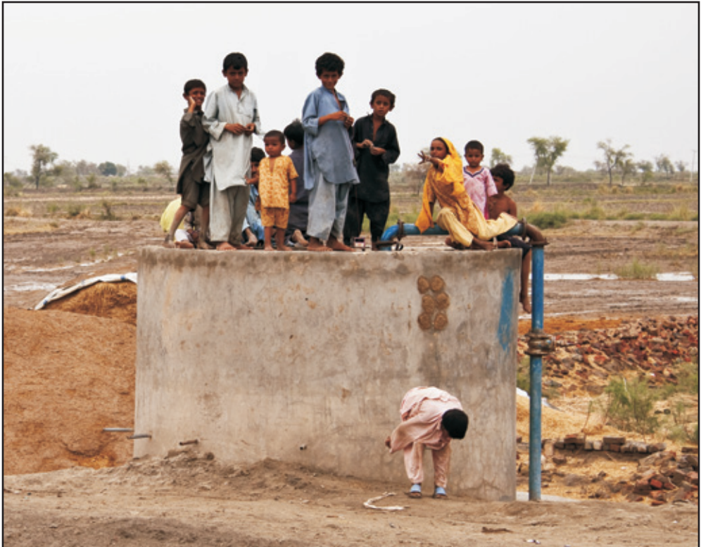
Construction of water supply system on village common land in Jacobabad, Sindh, Pakistan
